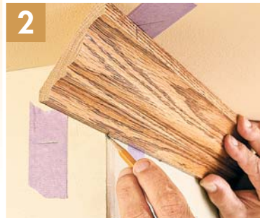
2 ▲ Establish Miter Angle To establish the miter angle, mark the bottom edge of each molding where it meets the wall, and the top where it aligns with the crosshair.
