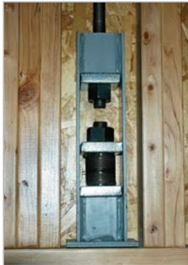
Previous Anchor Tiedown System
